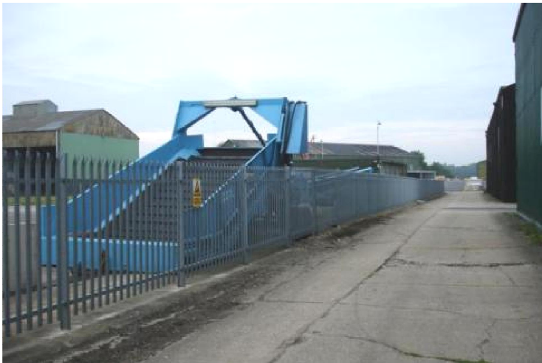
Insert 14.15 - View from Eye Airfield Industrial Park showing the remains of the north-west/south-east runway (HA31), facing north-west
