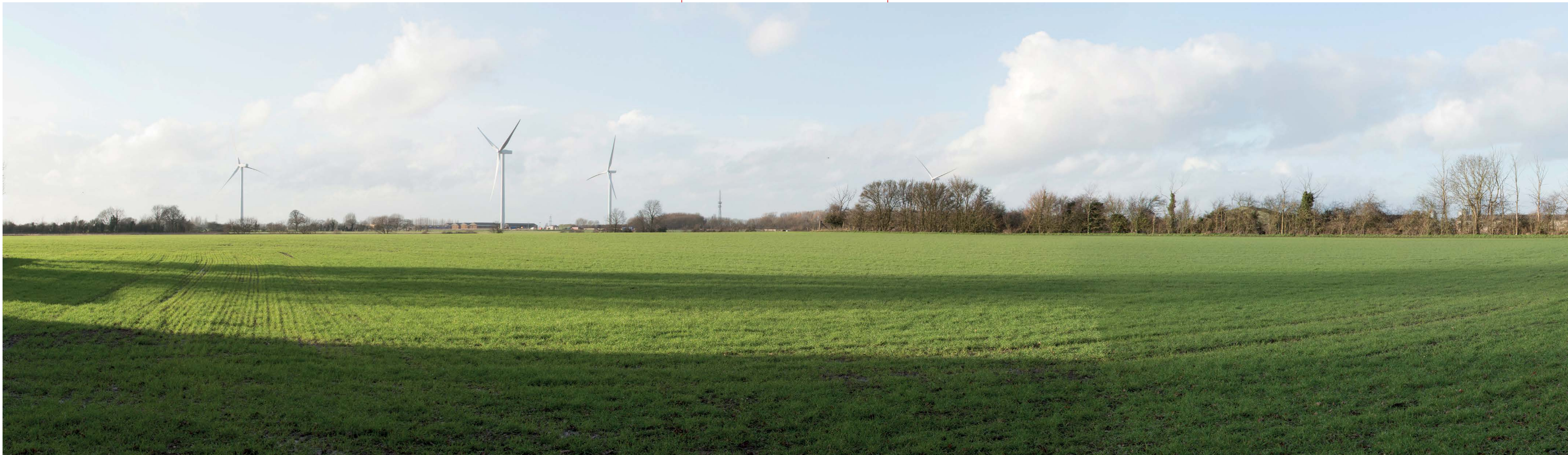
Power Generation Plant
