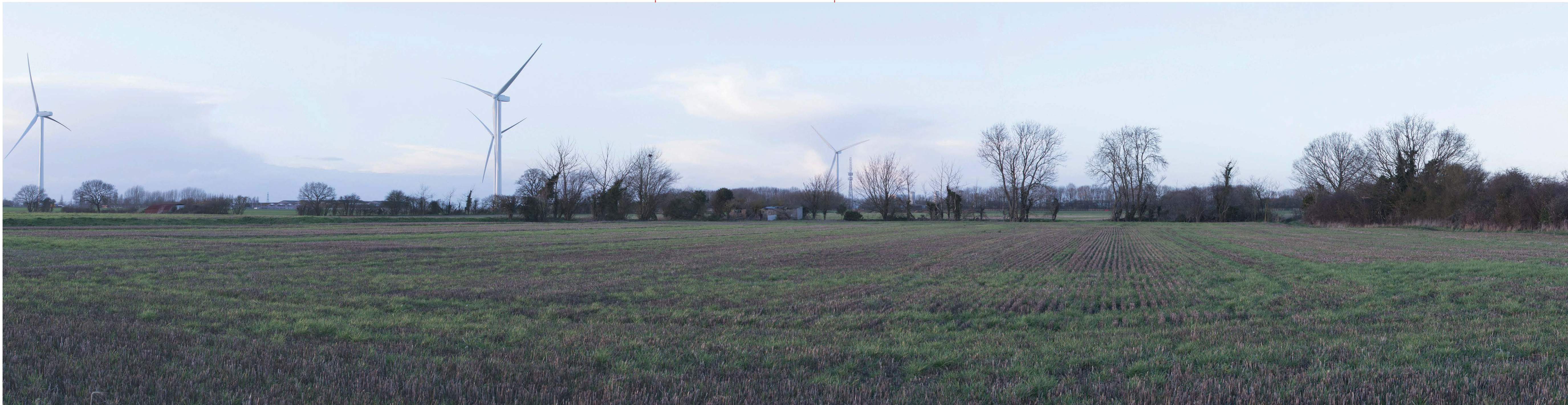
Power Generation Plant
