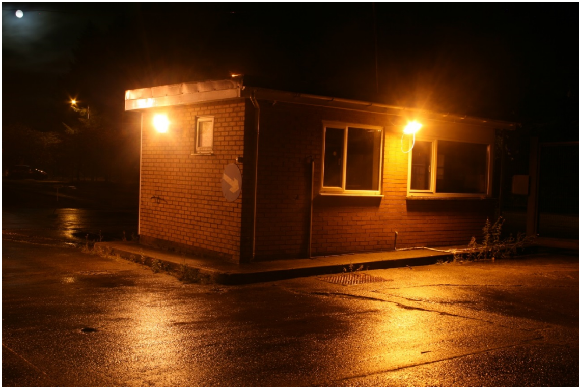
Figure 0.9: North-east corner of Security Bldg
