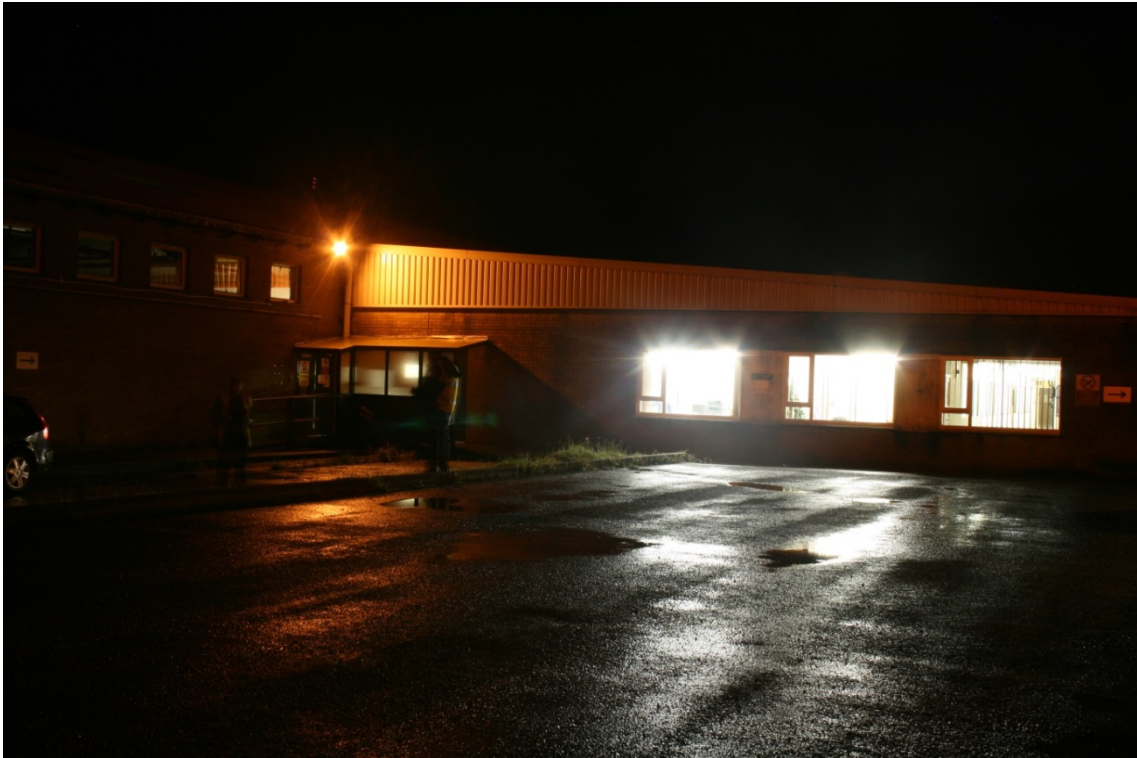
Figure 0.10: Security Light type B1 on South side of Bldg 1, near reception
