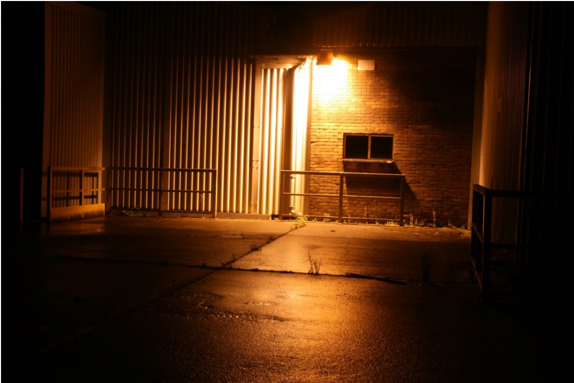
Figure 0.12: Type A light on north west corner of Bldg. 1 Figure 0.13: Type A lighting at south-west corner of Bldg 1
