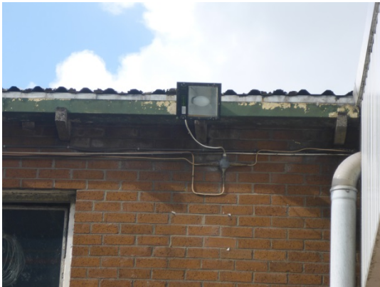
Figure 0.2: Type B1, near reception, south side of Bldg. 1
