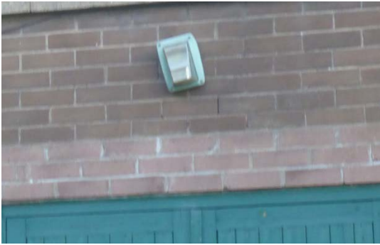
Figure 0.7: Type F located on south site of Bldg. 1
