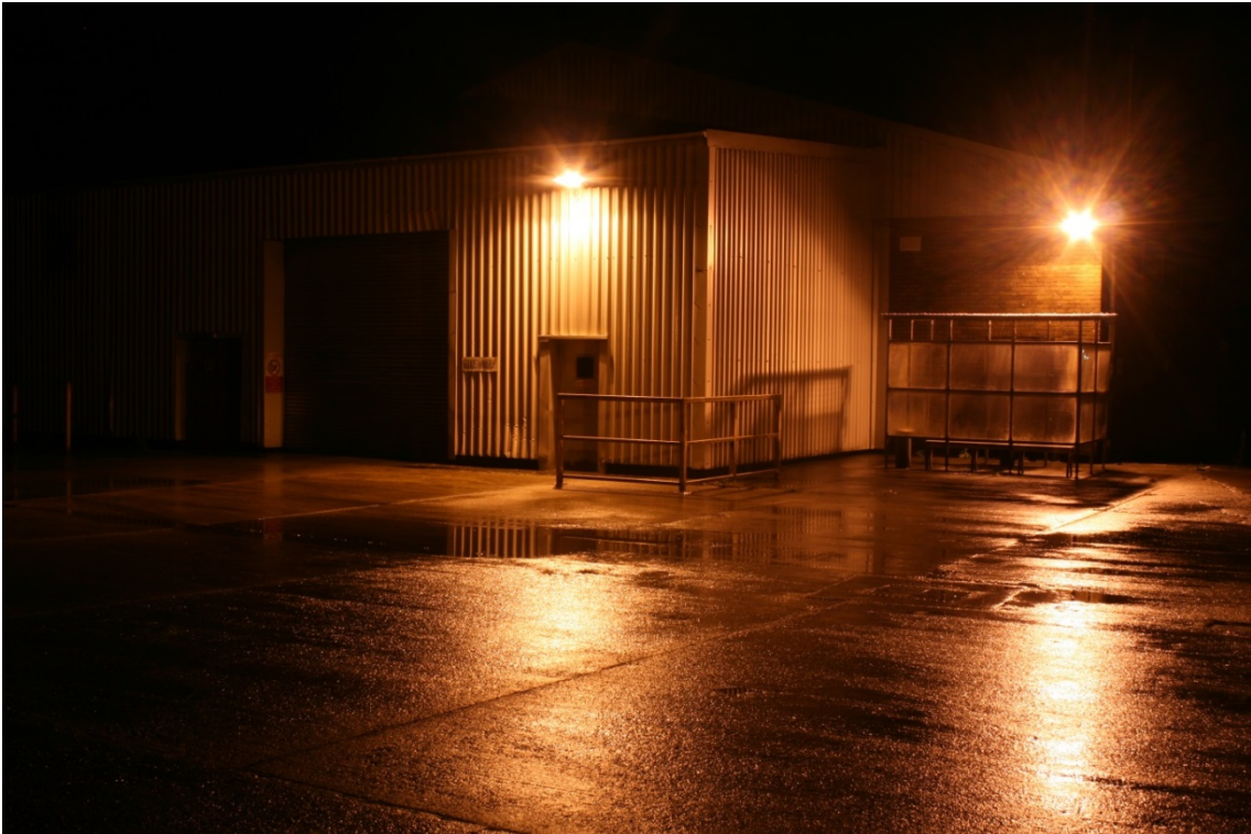
Figure 0.11: Type A and B light on south west corner of building 1
