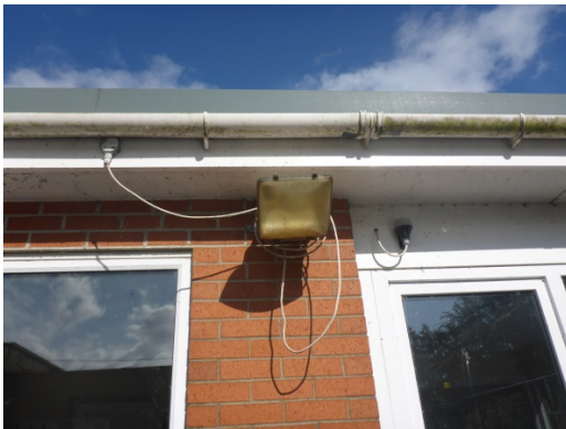
Figure 0.4: Type C, located on north side of Security Building (Gate 1)
