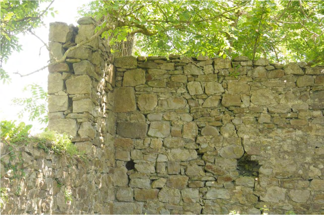
Photograph 18: Building 11 – Wall structure.
