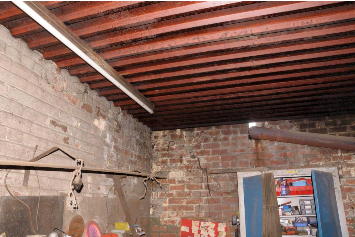
Photograph 12: Building 8 – ground floor.
