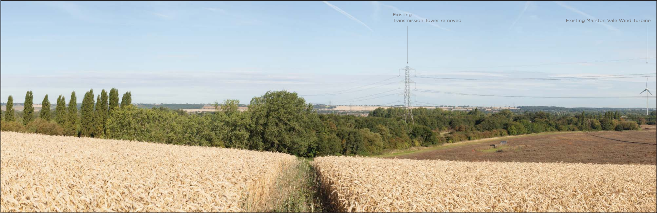
Existing baseline view from Country Park Access (72 degrees horizontal field of view, 32 cm viewing distance). View direction 317 - 29 degrees.
