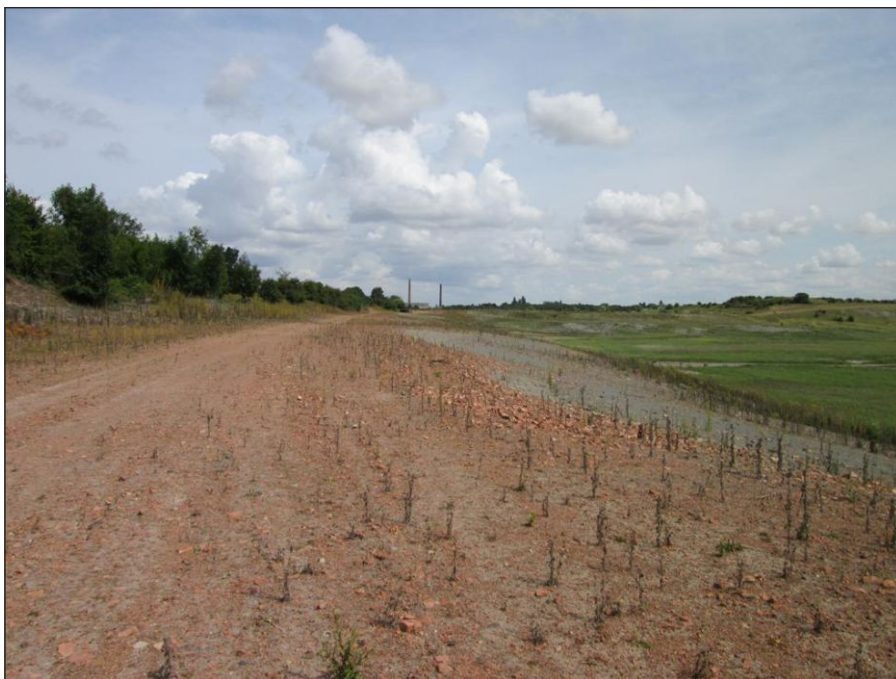
Plate 2 - Location of proposed access road looking north
